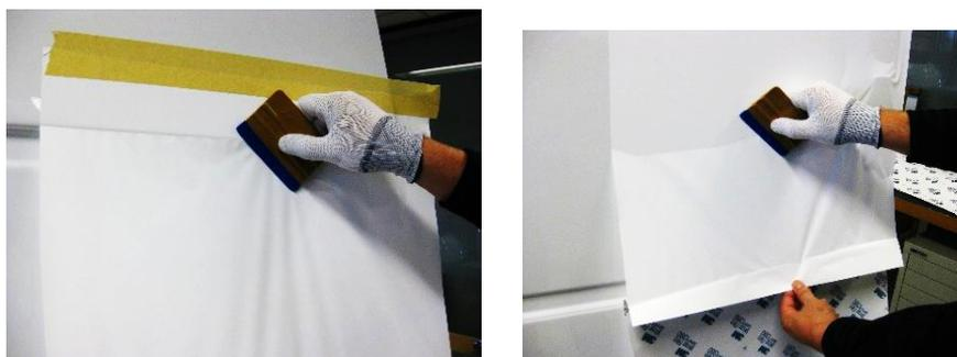
Apply the film manually or with appropriate tools on the recessed areas. Beside manual application, specially developed hand-rollers can be used for the application of the film into recessed areas. The hand-rollers (3M™ Roller S and L) allow the film to be applied with uniform, continuous pressure and low friction.
